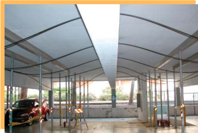
Unstressed external slab tendons
