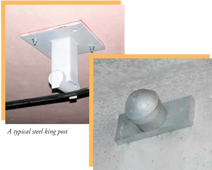
Galvanized anchor plate, barrel anchor and cap
