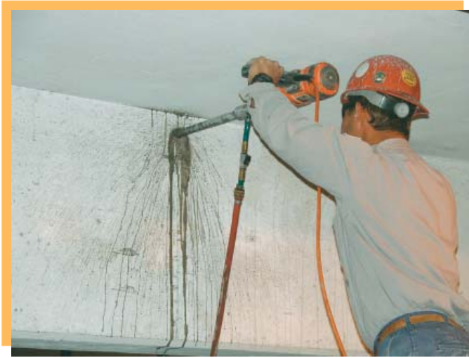
Coring through an existing beam
