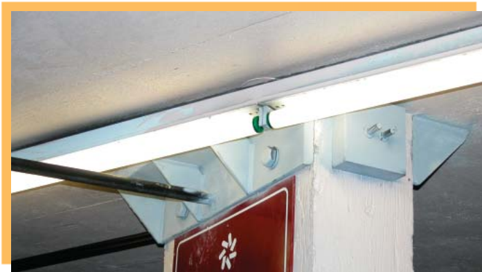
Anchoring at a column
