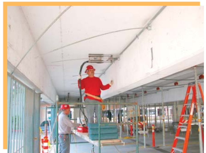
Stressing external tendons in an existing structure
