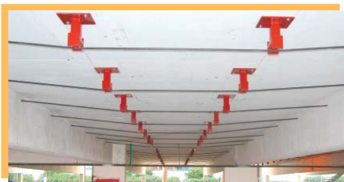
Final stressed condition of external slab tendons
