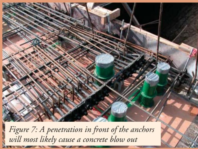
Figure 7: A penetration in front of the anchors will most likely cause a concrete blow out
