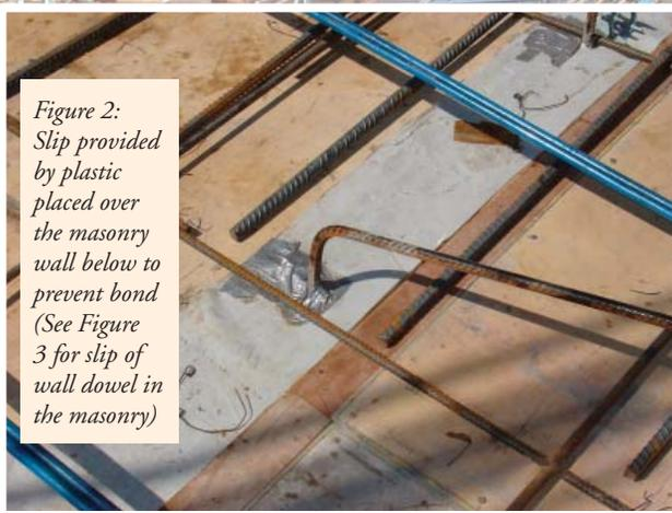
Figure 2: Slip provided by plastic placed over the masonry wall below to prevent bond (See Figure 3 for slip of wall dowel in the masonry)
