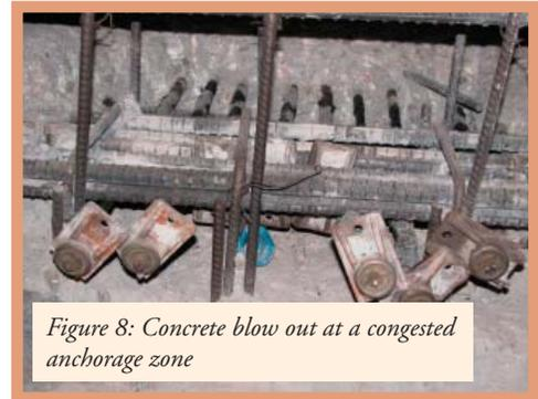
Figure 8: Concrete blow out at a congested anchorage zone
