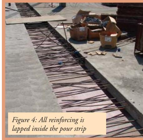
Figure 4: All reinforcing is lapped inside the pour strip
