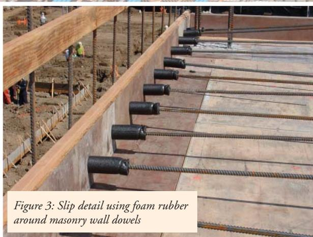
Figure 3: Slip detail using foam rubber around masonry wall dowels
