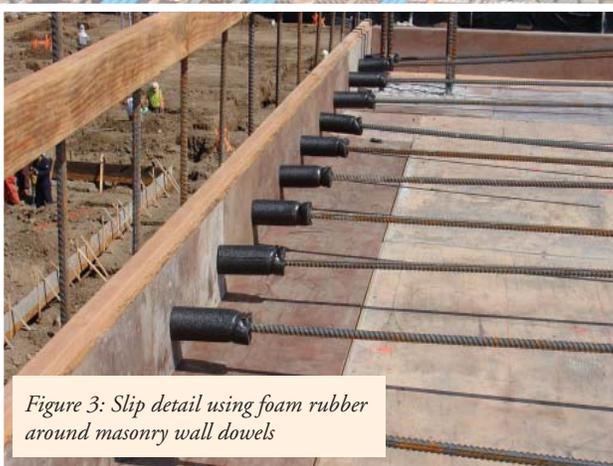
Figure 3: Slip detail using foam rubber around masonry wall dowels
