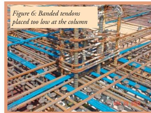
Figure 6: Banded tendons placed too low at the column
