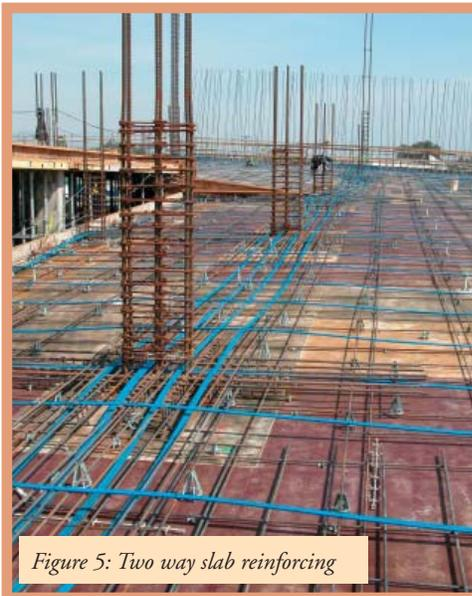
Figure 5: Two way slab reinforcing
