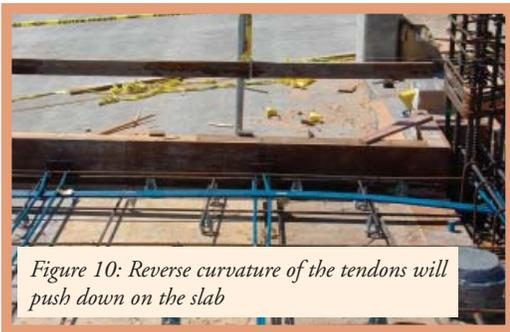
Figure 10: Reverse curvature of the tendons will push down on the slab
