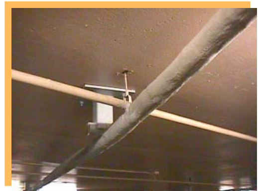
Fireproofing on grounded external tendons
