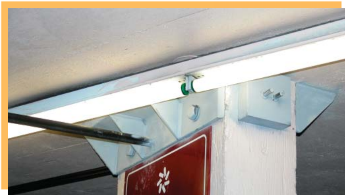
Anchoring at a column
