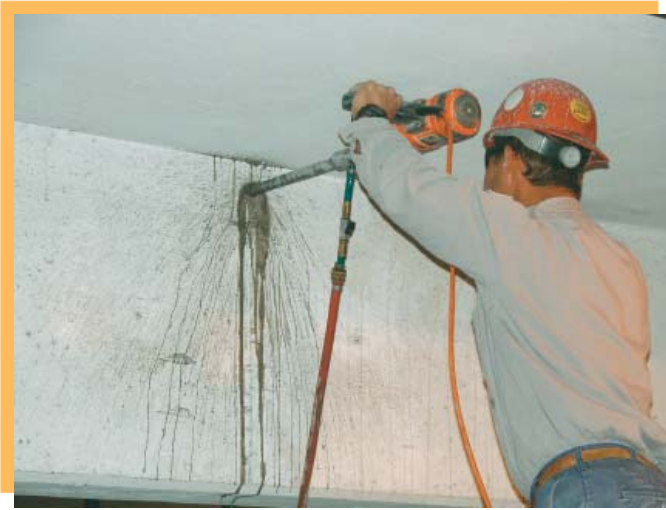
Coring through an existing beam
