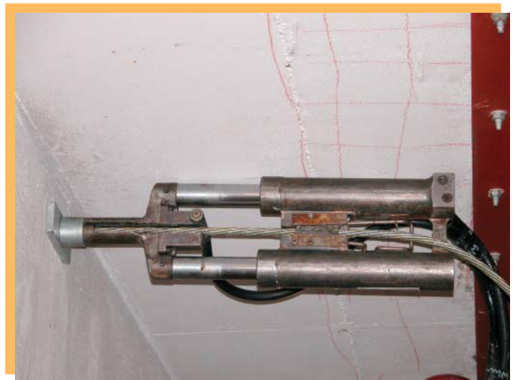
Close-up of the jack stressing the tendons
