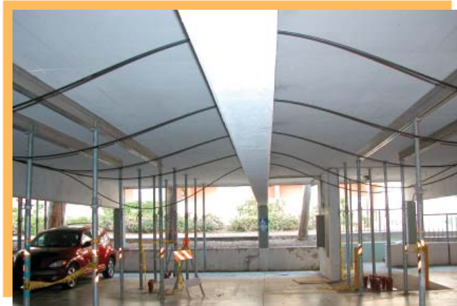
Unstressed external slab tendons
