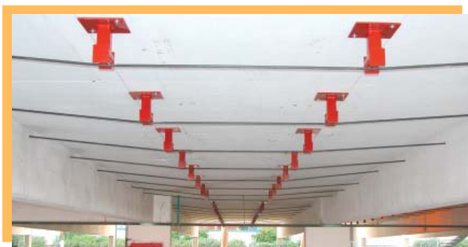
Final stressed condition of external slab tendons
