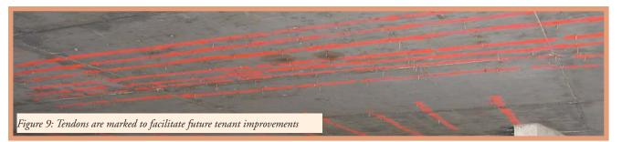
surface. I have personally used a \$40 metal detector and located tendons inside a 12-inch wide beam. For new office buildings where tenants frequently change, we recommend marking one side of the slab so that future tenants will know exactly where the strands and anchors were placed (*Figure 9*).
