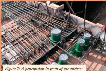
Figure 7: A penetration in front of the anchors will most likely cause a concrete blow out
