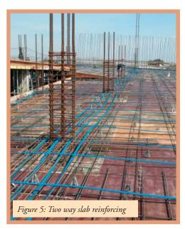
the entire tributary width will have a reduction. This is the closest way to achieve equal strength in both directions without additional strands or rebar.
