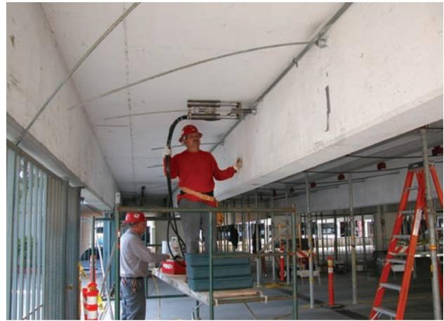
Fig. 13 – Stressing the Galvanized Tendons
