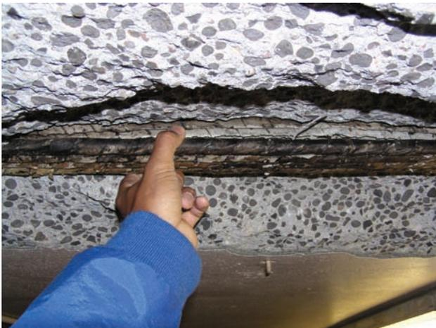
Fig. 6 – Broken Tendons Being Moved By Hand
