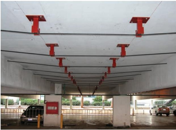
Fig. 10 – Double Harped External Post-Tensioning in a One-Way Slab
