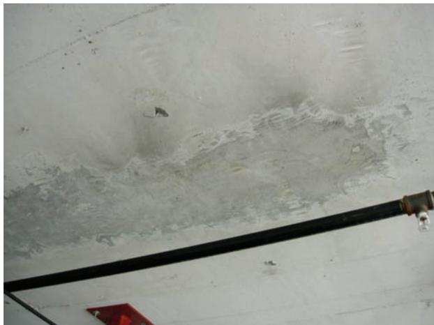
Fig. 8 – Patched Concrete
