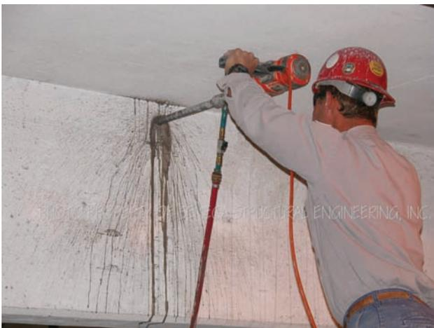
Fig. 12 – Drilling Through an Existing Post-Tensioned Beam
