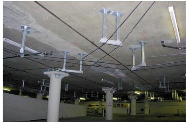
Fig. 14 – A Double Harp Two-Way EPT System
