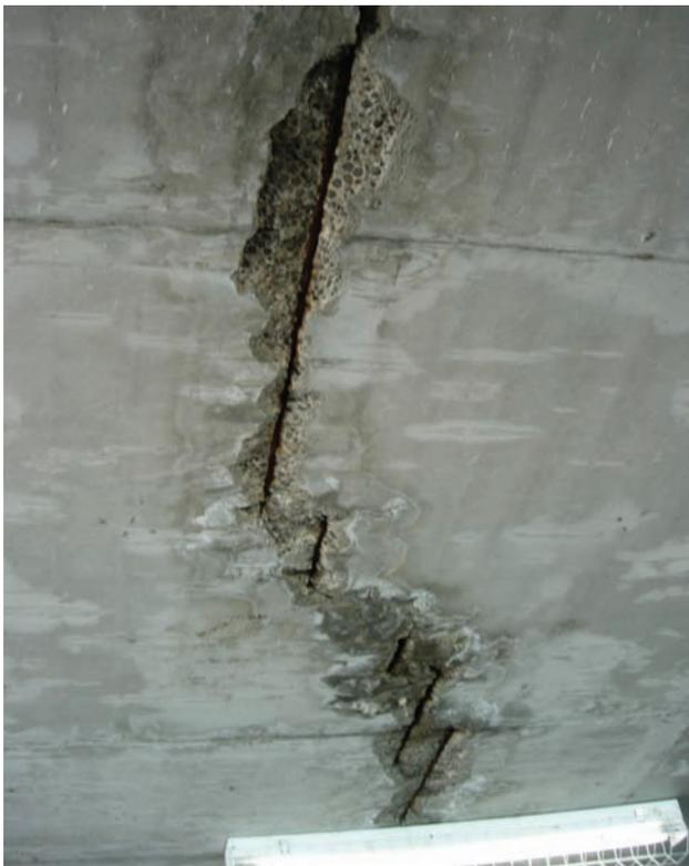
Fig. 3 – Water Staining, Rust and Efflorescence at Corroded Reinforcing
