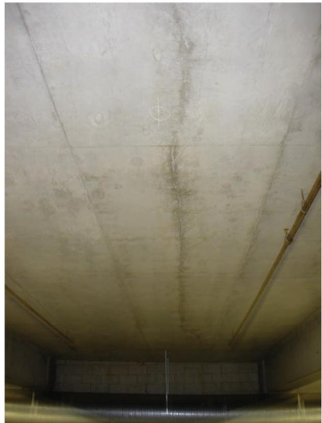
Fig. 7 – Full Length Mid-span Crack Parallel to Beams
