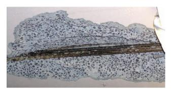
Fig. 2 – Corroded Tendons
