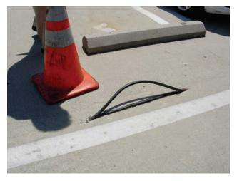
Fig. 4 – A Broken Tendon in Extruded Sheathing
