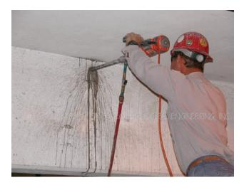
Fig. 12 – Drilling Through an Existing Post-Tensioned Beam
