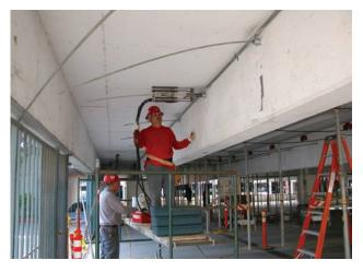
Fig. 13 – Stressing the Galvanized Tendons
