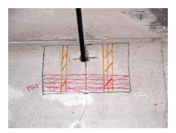
Fig. 11 – X-Ray Markings on a Existing Post-Tensioned Beam
