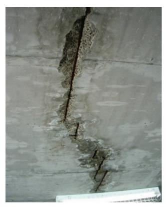
Fig. 3 – Water Staining, Rust and Efflorescence at Corroded Reinforcing
