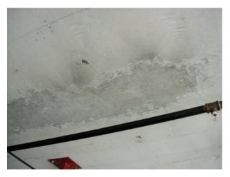
Fig. 8 – Patched Concrete
