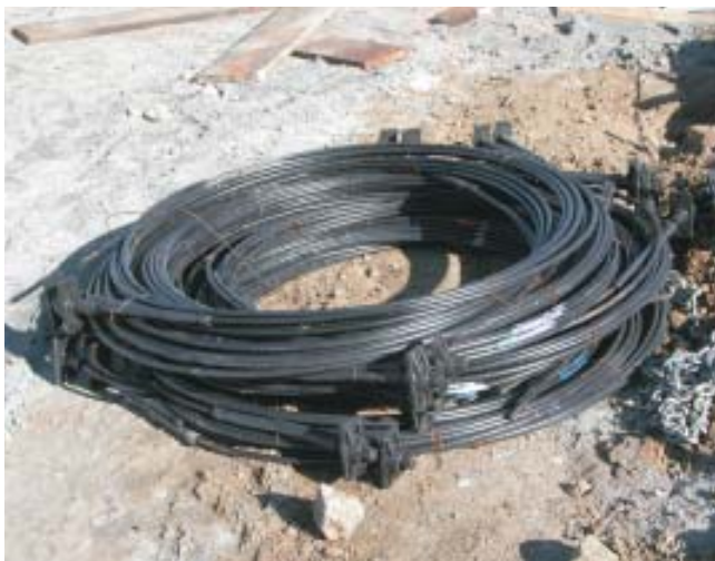
Figure 4. The plastic-coated tendons arrive at the site cut to length, with one anchor plate already wedged in place (left). The preattached dead-end anchor is nailed to the form board half the slab thickness from its top edge, and a U-shaped steel backup bar is wired to the anchor to help distribute the eventual tensioning pressure over a wider area of the slab edge (right). The thick sleeve at the end of the tendon is designed to protect the cable and fitting from corrosive soils present on this site; in noncorrosive soils it could be omitted.
