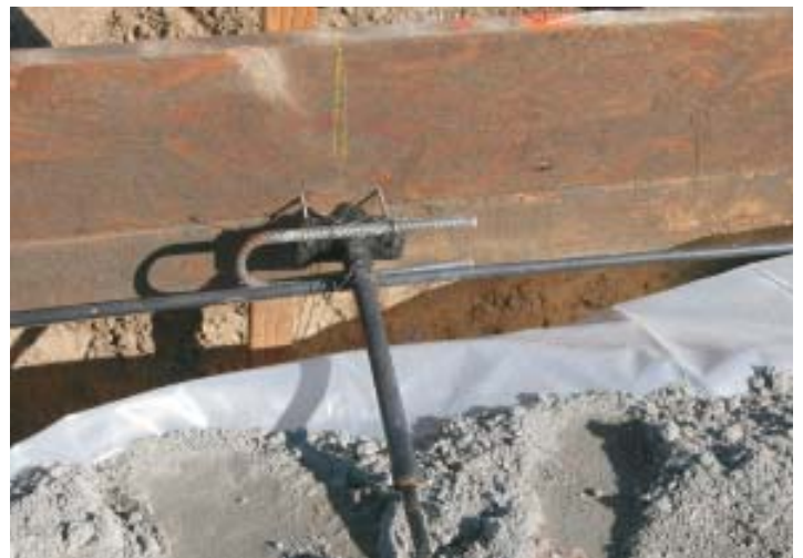
Figure 4. The plastic-coated tendons arrive at the site cut to length, with one anchor plate already wedged in place (left). The preattached dead-end anchor is nailed to the form board half the slab thickness from its top edge, and a U-shaped steel backup bar is wired to the anchor to help distribute the eventual tensioning pressure over a wider area of the slab edge (right). The thick sleeve at the end of the tendon is designed to protect the cable and fitting from corrosive soils present on this site; in noncorrosive soils it could be omitted.
