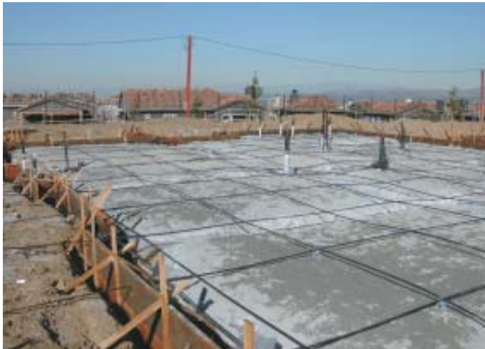
Figure 6. Tendons are supported by plastic chairs and wired together where they intersect (above). In some limited areas, such as this inside corner next to a garage door opening, conventional rebar provides added resistance to cracking (right).
