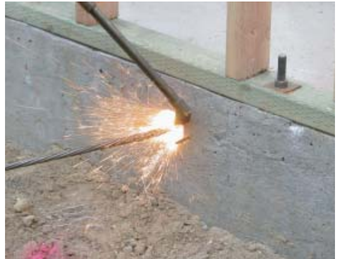
Figure 8. Tendons are tensioned with a portable hydraulic ram. The round gauge on the hydraulic power unit lets the operator know when the required amount of force has been reached (above left). After the newly tensioned cables have been locked in position with steel wedges, the protruding ends of the cables and the nails used to fasten the cast-iron anchors to the forms are cut off with an acetylene torch (above right). The remaining pockets will later be filled with grout (left).
