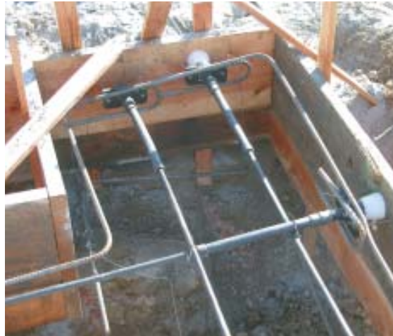
Figure 6. Tendons are supported by plastic chairs and wired together where they intersect (above). In some limited areas, such as this inside corner next to a garage door opening, conventional rebar provides added resistance to cracking (right).
